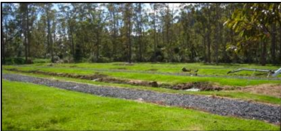
Figure 23: Matarangi WWTP Diffusion Beds
